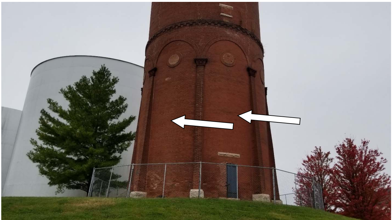
Photograph #2 – Photograph of approximate location of lateral bowing observed in exterior masonry walls. The bowing was observed around the perimeter of the tower at approximately 15' +/- above grade
