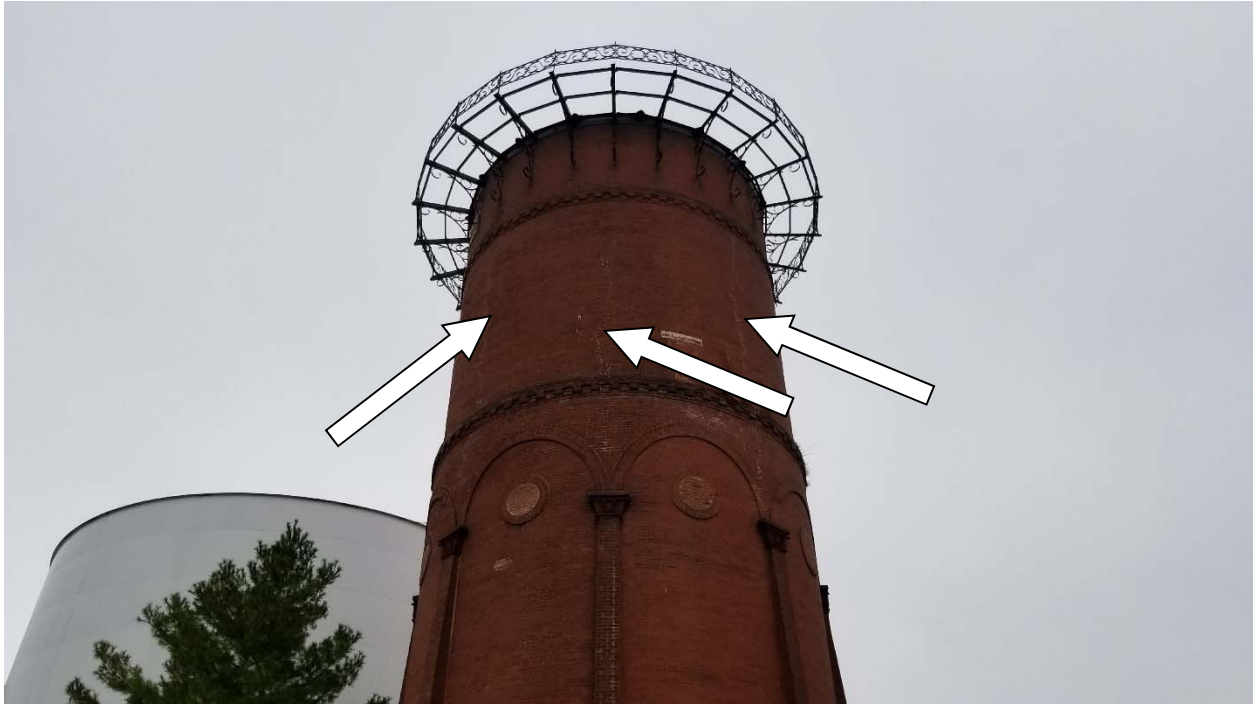
Photograph #1 – Photograph of vertical cracks on exterior surface of brick masonry around perimeter of water tower
