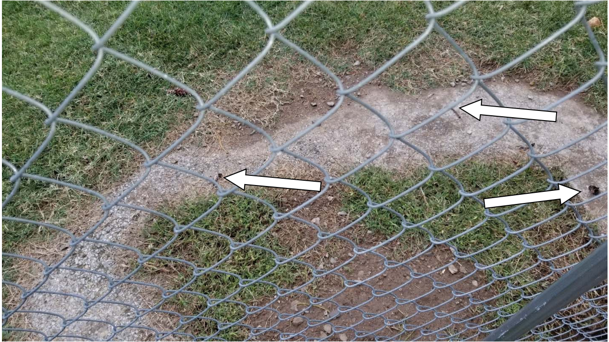
Photograph #11 – Photograph of nails, nuts, bolts, and other metal hardware on ground outside of fence at base of tower. The hardware appeared to have fallen from the wrought iron handrail and platform located at the roof of the tower
