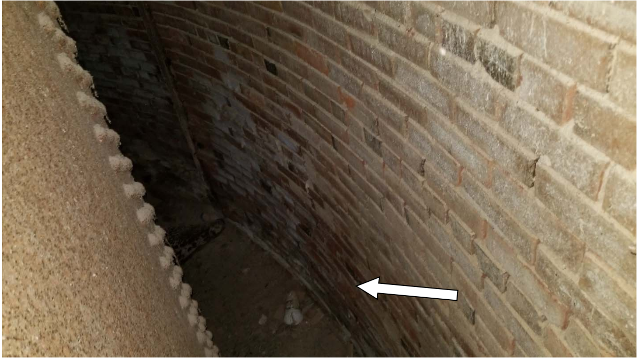
Photograph #7 – Photograph of deteriorated mortar joints on interior surface of tower wall. Lateral bowing was also observed at several locations on the interior surfaces of the tower wall
