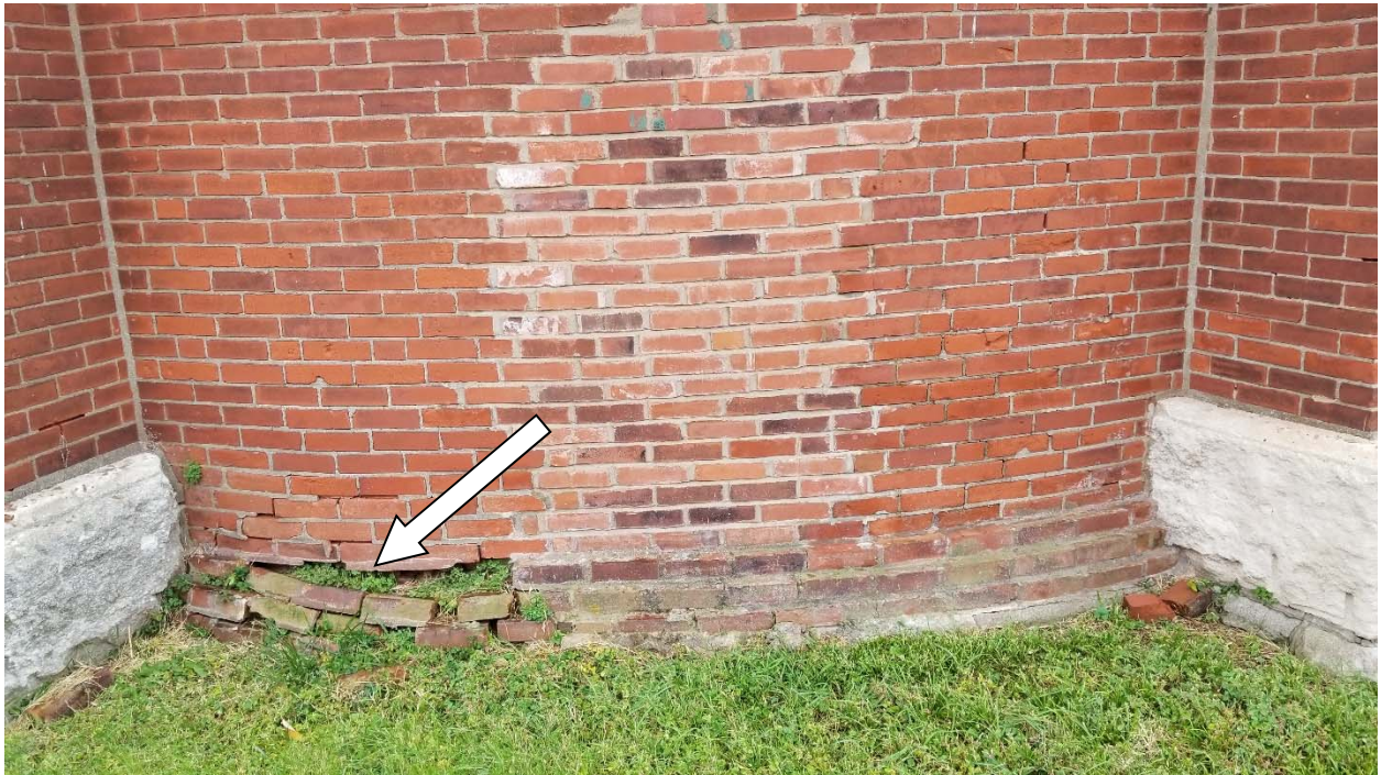
Photograph #5 – Photograph of loose bricks at base of tower
