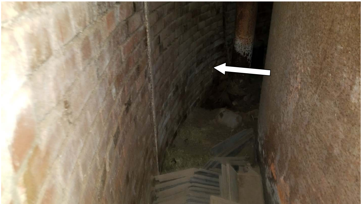
Photograph #8 – Photograph of loose bricks on interior surface of tower wall
