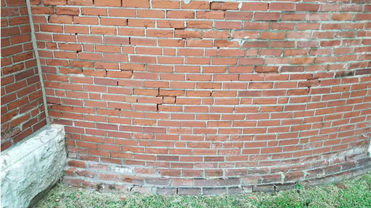
Photograph #3 – Photograph of spalled bricks and missing mortar on exterior surface of tower
