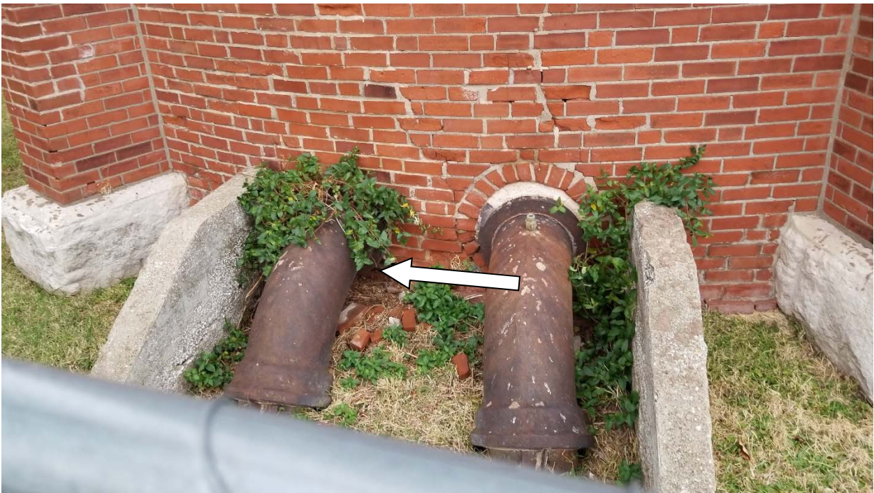
Photograph #4 – Photograph of loose bricks at base of tower
