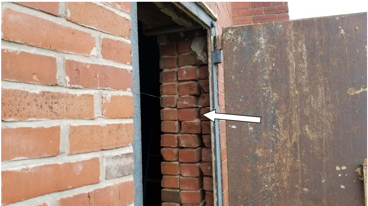
Photograph #6 – Photograph of loose bricks at edge of door opening. The mortar on the interior surfaces of the tower walls was deteriorated and large voids between the bricks were observed
